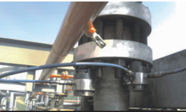
ACCURATE TENSIONING SERVICES
